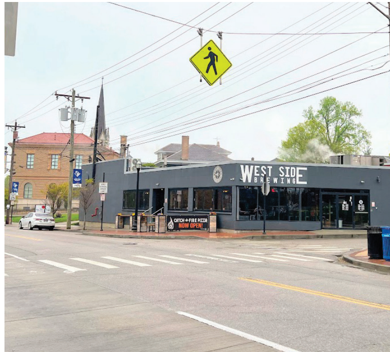
West Side Brewery and Madcap along Harrison Avenue
